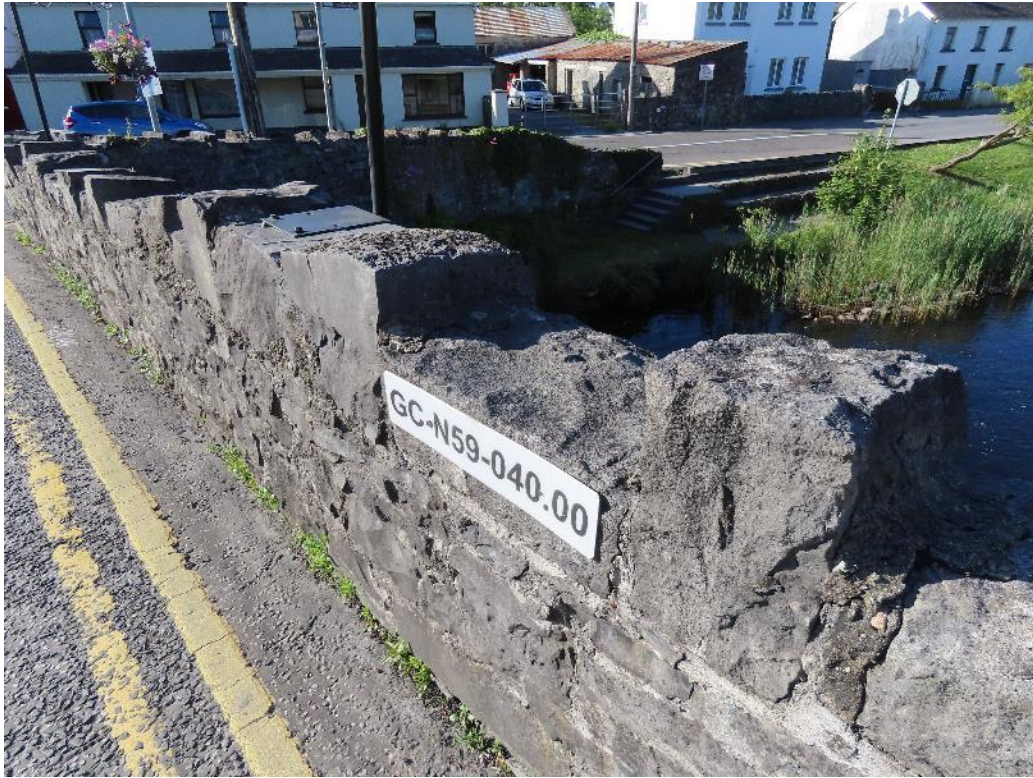
Photo 28 – downstream parapet wall of existing bridge
