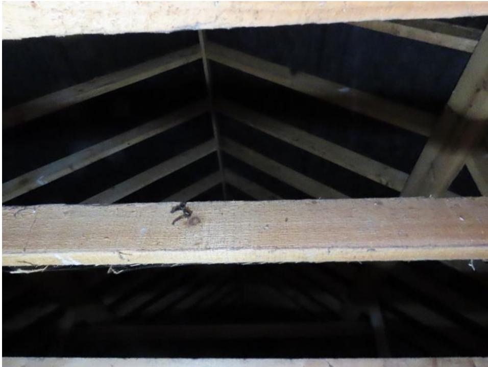
Photo 19 – roof lined internally with bitumen felt
