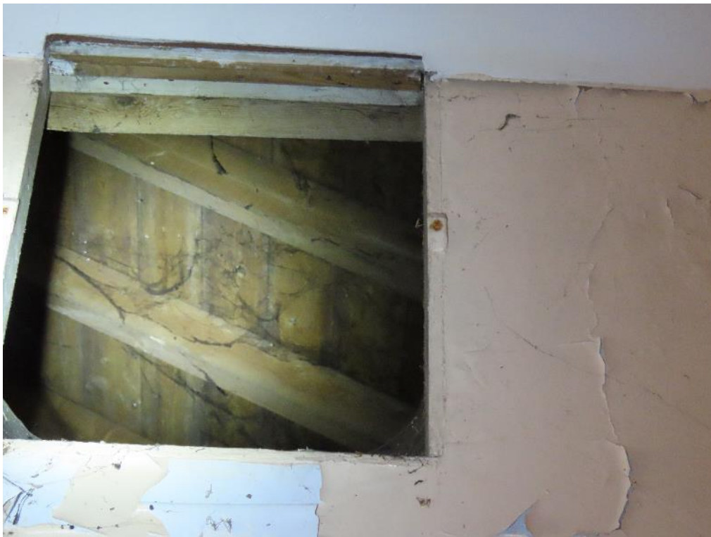
Photo 16 – hatch to attic space in eastern side of building. Roof tiles lined internally with wooden sarking boards
